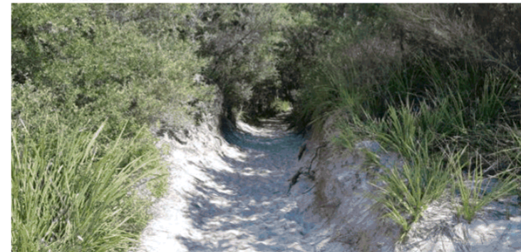
Figure 5-1 – Erosion at base of track (Hyams Beach). Consider reorienting track so it doesn't face south and is more perpendicular to the beach, and consider installation of timber sleepers at base to reduce the effects of this erosion.
