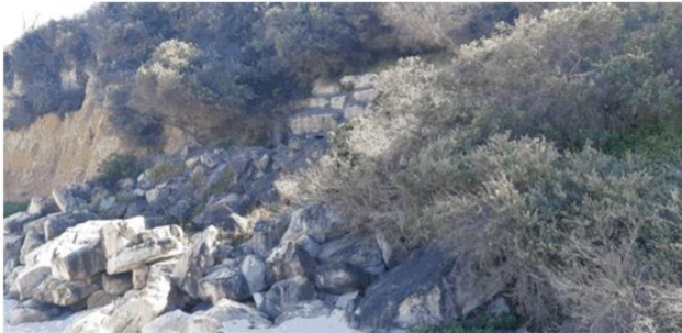
Nelson Beach – slope stability, stormwater outflow
