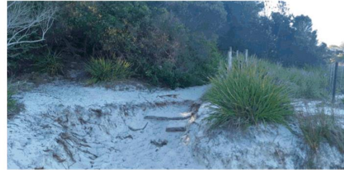
Hyams Beach – erosion of base of walkway
