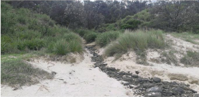
Path eroded by stormwater at Cunjurong Point
