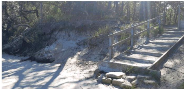
Myola – erosion of creek bank impacting on access
