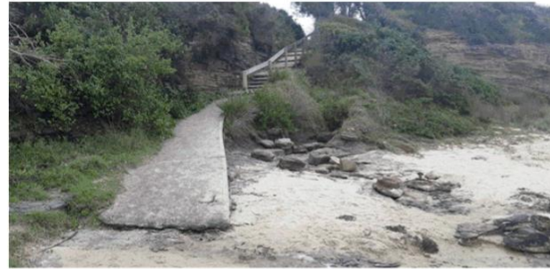
Berrara - Erosion due to runoff
