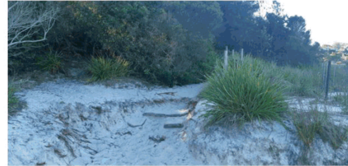
Figure 5-1 – Erosion at base of track (Hyams Beach). Consider reorienting track so it doesn't face south and is more perpendicular to the beach, and consider installation of timber sleepers at base to reduce the effects of this erosion.
