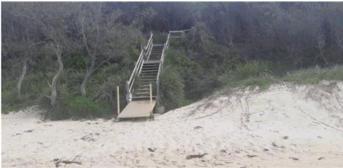
Undermined stairway affected by slope instability at Cunjurong Point
