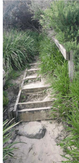
Damaged and overgrown stairway at Bendalong
