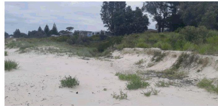
Collingwood Beach – stormwater erosion
