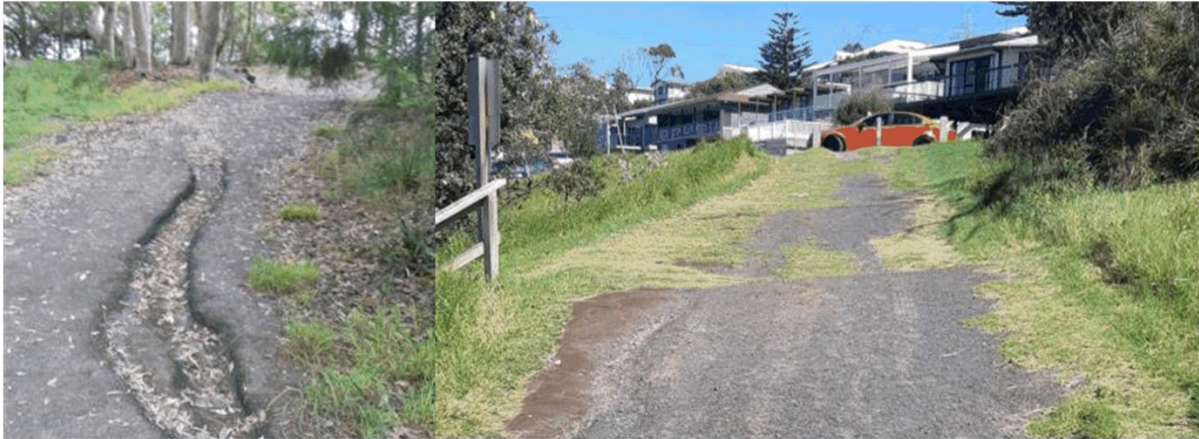
Figure 3-10 – Example of drainage control "hump" in gravel path, Mollymook Beach, March 2021.
