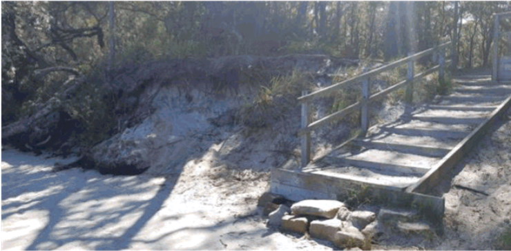
Figure 3-39 – Severe bank erosion at Moona Moona Creek adjacent to timber stairway (February 2021)
